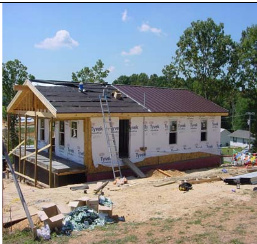
Figure 29. Roof drainage plane under the raised metal roof. (See http://www.englertinc.com/roofing-panels.aspx?Page=7 ).
