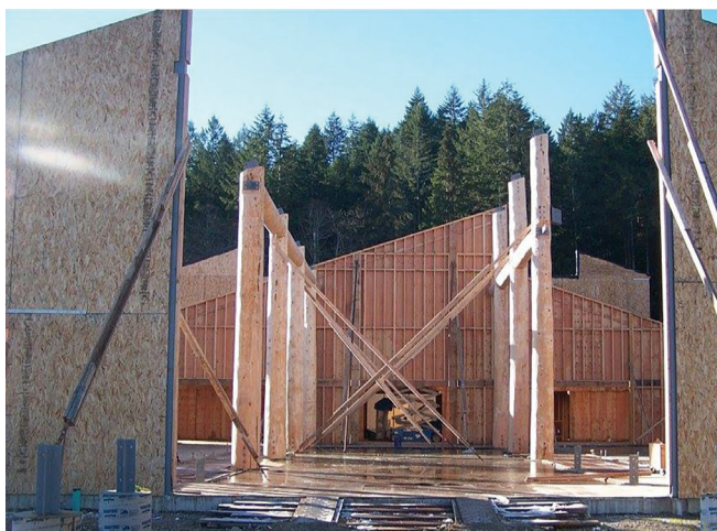
Skokomish Community Center, Shelton WA
