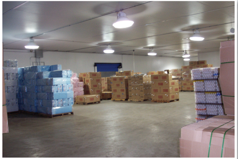
Interior freezer and suspended ceiling.
